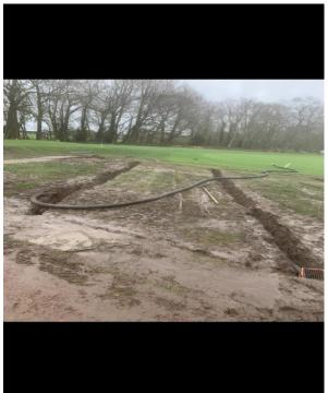
To stop the water from gathering, we installed a flood grid at the end of one of our drainage laterals, in the low spot near the Oak, to stop water building up there. The image on the left here shows how much water was being held here and the image on the right, shows a side profile of what the water was facing to get through to the pipes.
